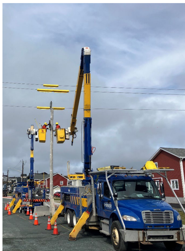
Newfoundland Power crews performing a transmission pole replacement in the St. John's region.
