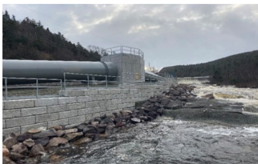
Petty Harbour hydroelectric plant penstock and forebay dam viewed from the trailrace.
